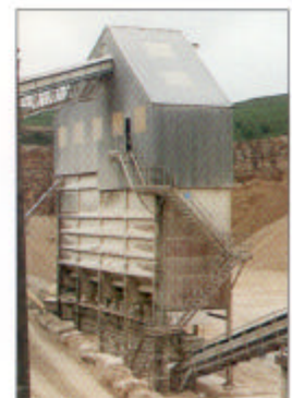
Quarry screen house. Roadstone.
