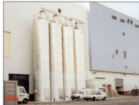
Vegetable oil storage at food manufacturing plant.
